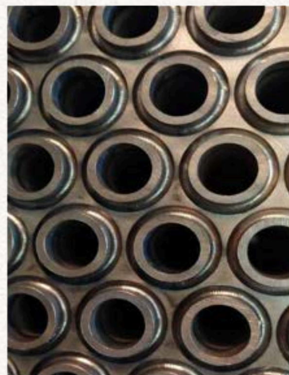
Figure 3 Orbital tube to tube sheet-Root weld
