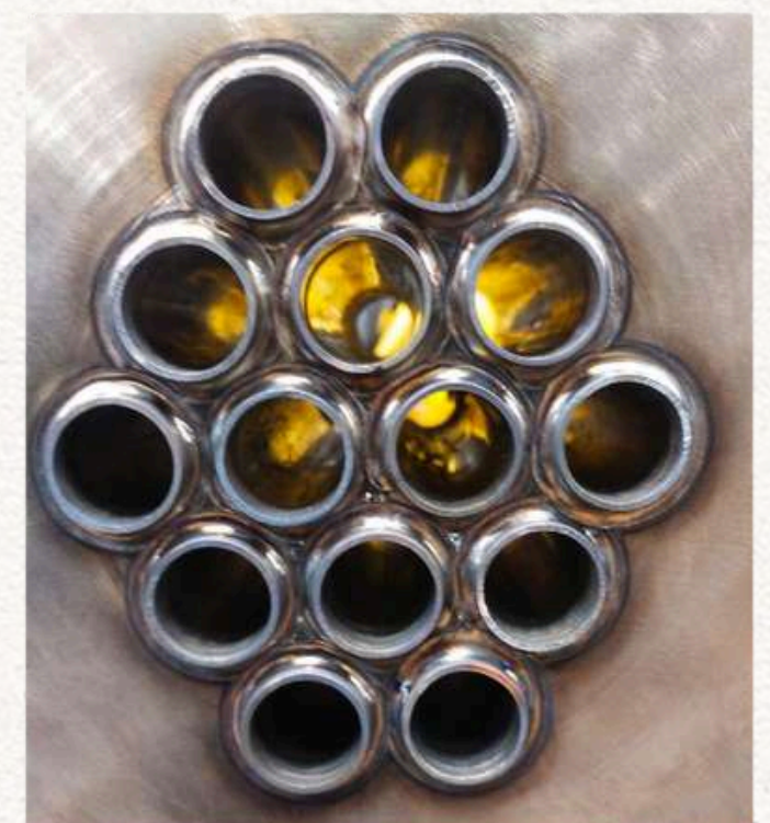
Figure 3 Orbital tube to tube sheet-Completed weld
